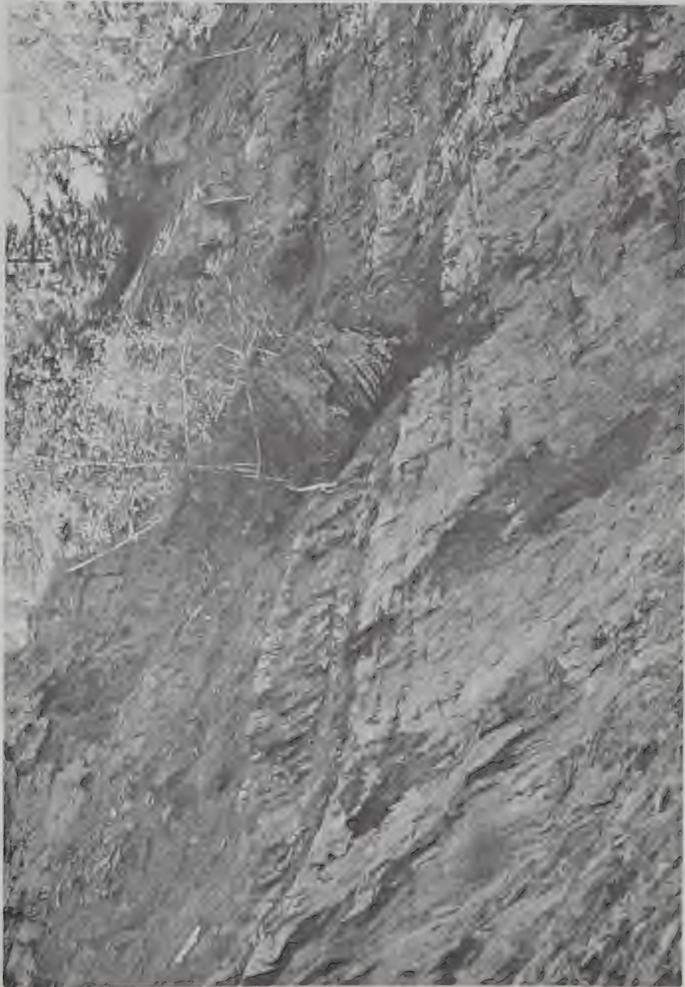
PLATE 3.3 Block Falls and Exfoliation Scars on Slope #7 (Appendix A)
